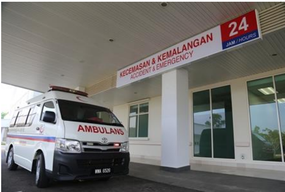
Fig. 2 Emergency entrance of Sultan Ahmad Shah Medical Centre (Source: https://kmihealthcare.com/ )
